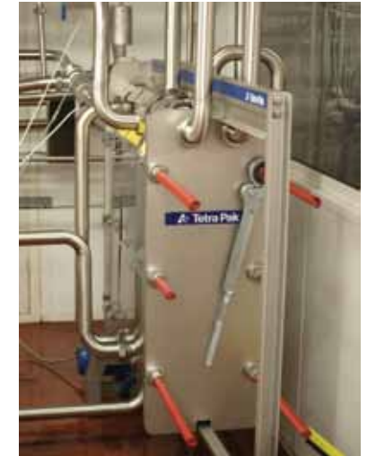
A new Tetra Plex plate heat exchanger provides a high level of heat recovery and is able to process fibrous liquids
